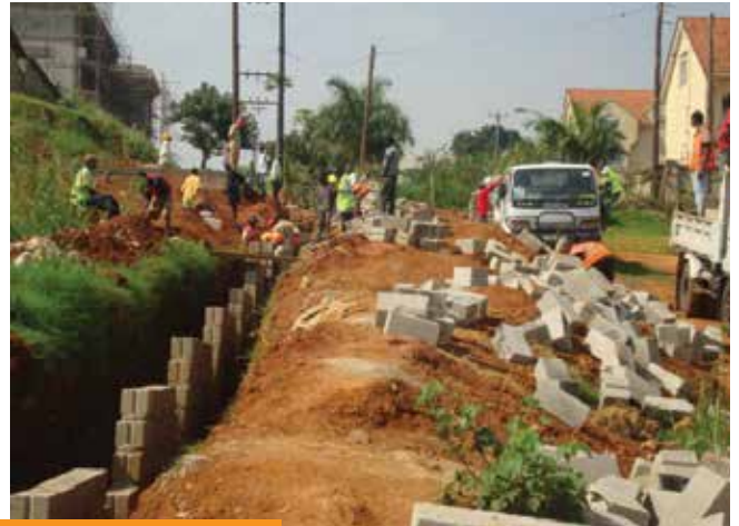
FOUNDATION CONSTRUCTION
